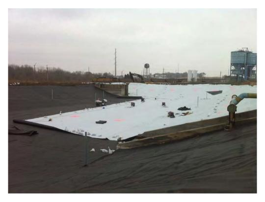
View of 16 oz geotextile in place and HDPE liner being placed.
