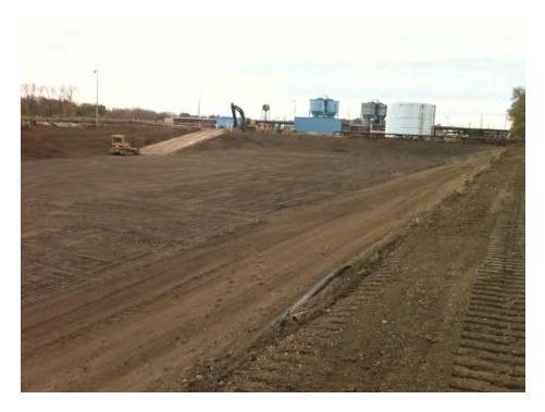
View of basin subgrade from the northwest corner of the basin facing southeast. Note concrete aprons and hypalon removed.
