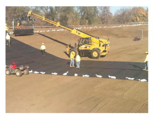
View of 16 oz geotextile being placed on the western slope and thermally bonded at the seams.
