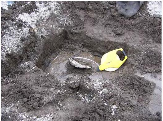
View of the uncovered leak in the bypass basin from the detection survey.
