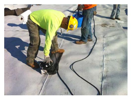
View of extrusion seaming vacuum testing.
